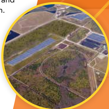
COMING SOON: SOLAR FARM II 13 MW
