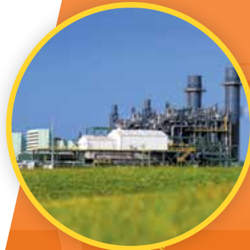
UNITS A & B NATURAL GAS 940 MW
