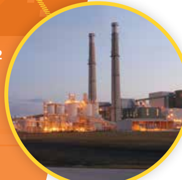
UNITS 1 & 2 COAL 940 MW
