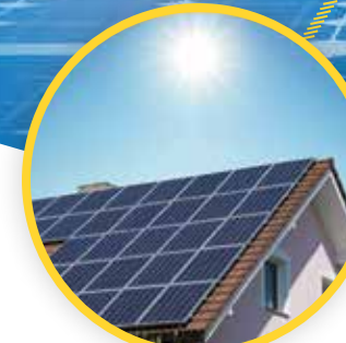
RESIDENTIAL ROOFTOP SOLAR
